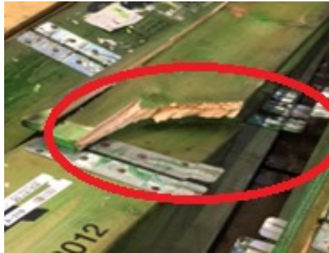
1. Repair, broken plank
