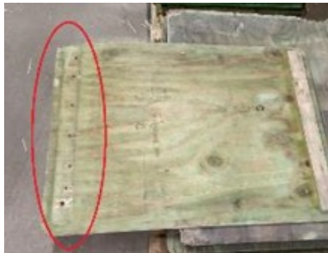
1. Repair, missing plank
