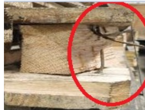
7. Repair, broken block
