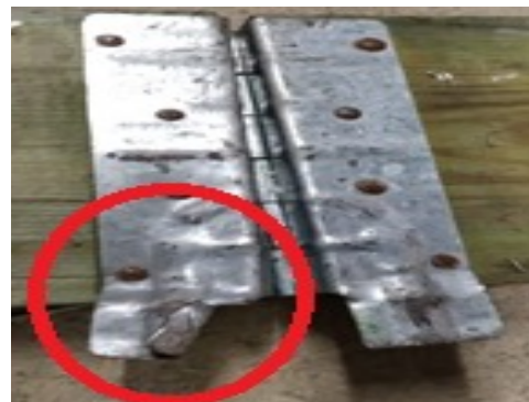
6. Repair, bent hinge
