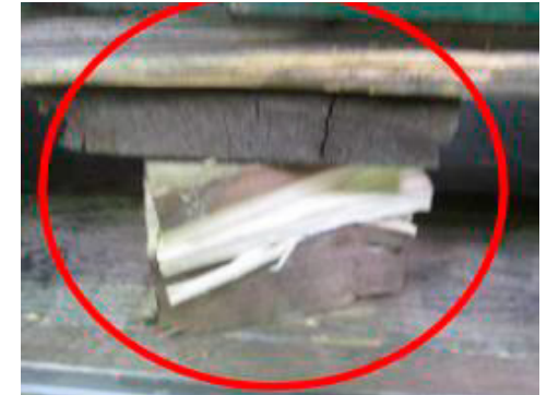
8. Repair, broken block
