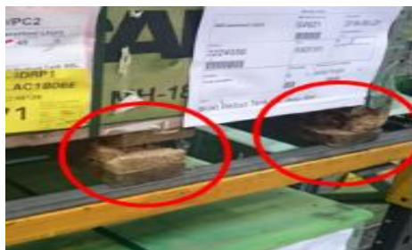
Broken, loose and/or missing Blocks
